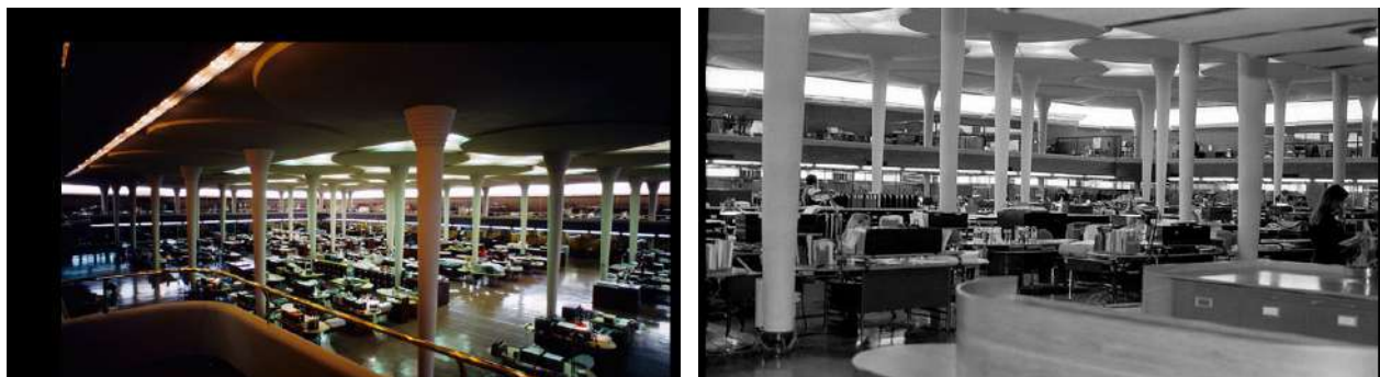
Рис. А.2 Johnson Wax Building. The open workspace is a half-acre wide and 21 feet in height. The Roof is supported by “mushroom columns” that is wide at the top and thins to nine inches at the bottom
